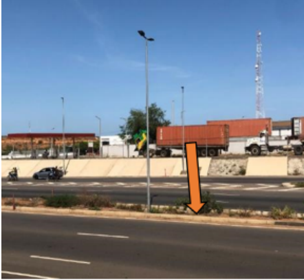
Figure 9: Refuge island without kerb ramp (TMI)
