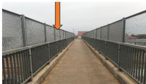
Figure 13: Disability pedestrian ramp enclosed by footbridge Ramp handrails on both sides (TMI)
