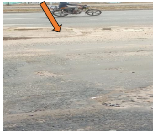
Figure 8: Refuge island with kerb ramp (TQI)
