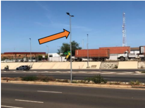
Figure 18: Streetlights at TMI
