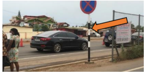
Figure 16: Signage at TMI in a relatively better state
