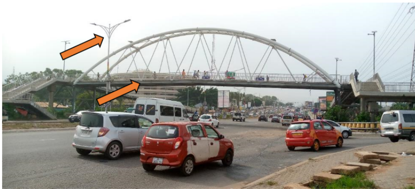
Figure 20: Footbridge and Streetlights at TQI
