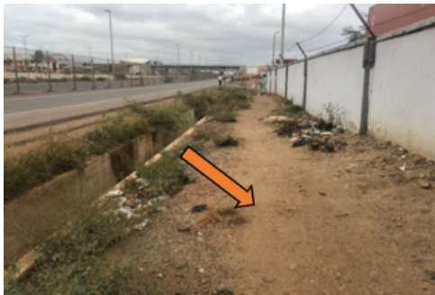
Figure 6: Unpaved Pedestrian Walkway with opendrains at TMI
