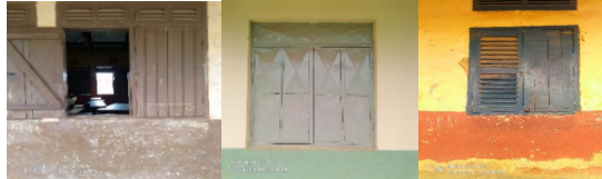
Figure 1: Variations of Casement fenestrations used in Public Basic Schools
