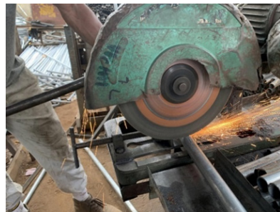
Fig 20: Measuring and cutting of the frame
