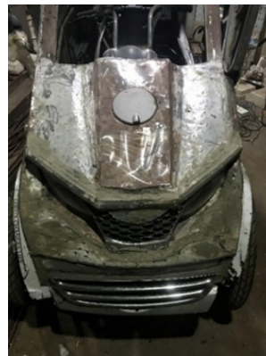
Fig 60: Applying fiber filler
