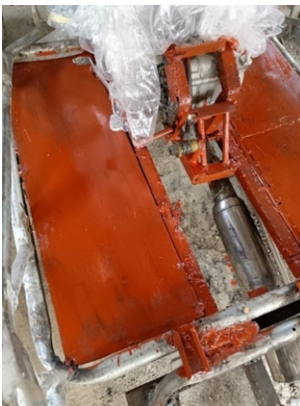
Fig 58: Application of red oxide onto all iron part
