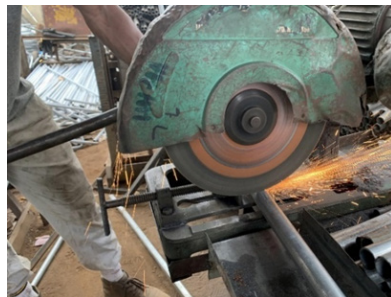
Fig 20: Measuring and cutting of the frame
