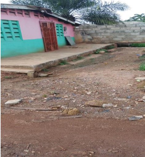
Figure 1: A picture of an African Independent church building causing sheet erosion
