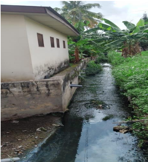
Figure 2: A picture of a church building causing water pollution and an unhealthy environment
