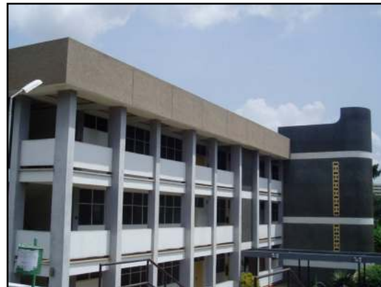
Plate 2: A building with roof parapet walls
