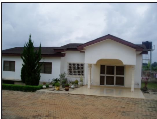
Plate 1 A building without roof parapet walls
