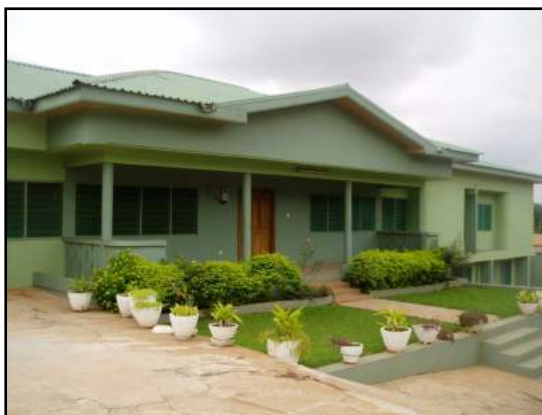
Plate7: A building with a redesigned roof, eliminating the concrete gutter altogether
